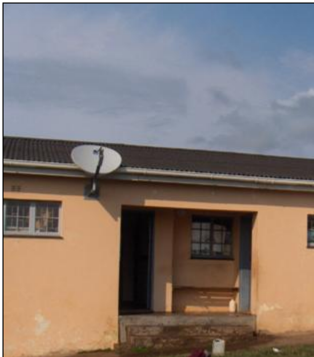
Figure 3.1: VSAT deployed at Mpume
