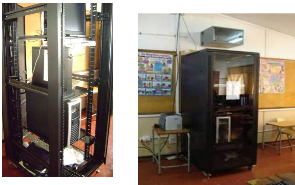
Figure 4.4: Equipment put in a lockable rack
