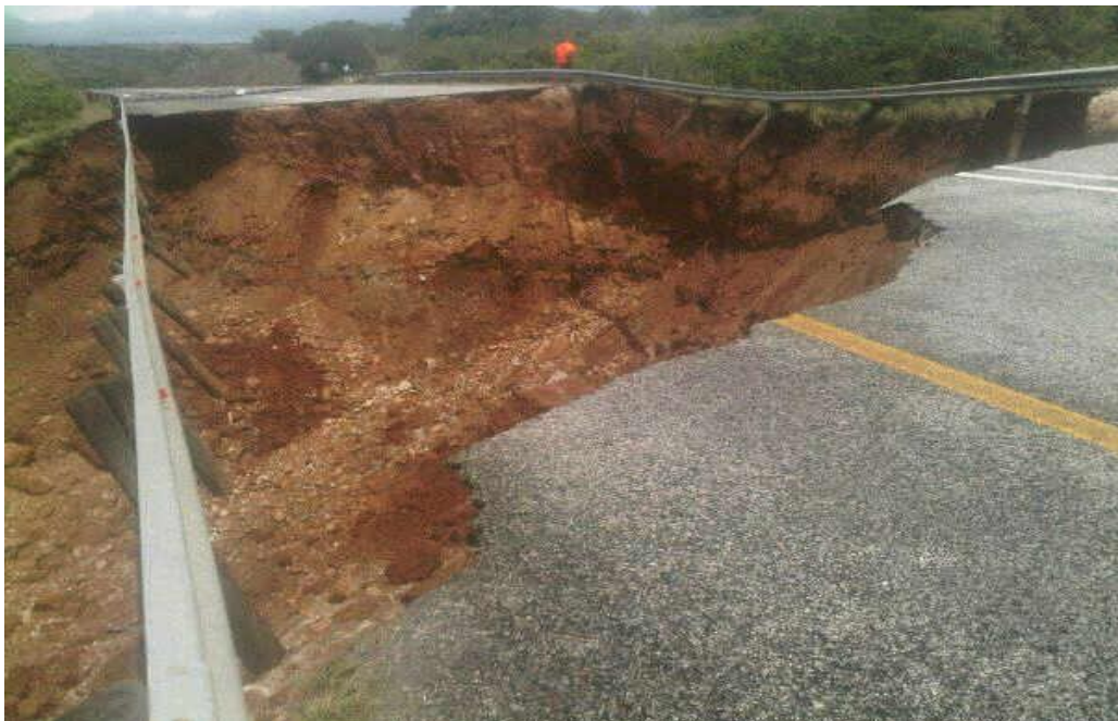
Fig. 2.7: Road erosion caused by wave and tide current at Port Elizabeth coast in 2012.
