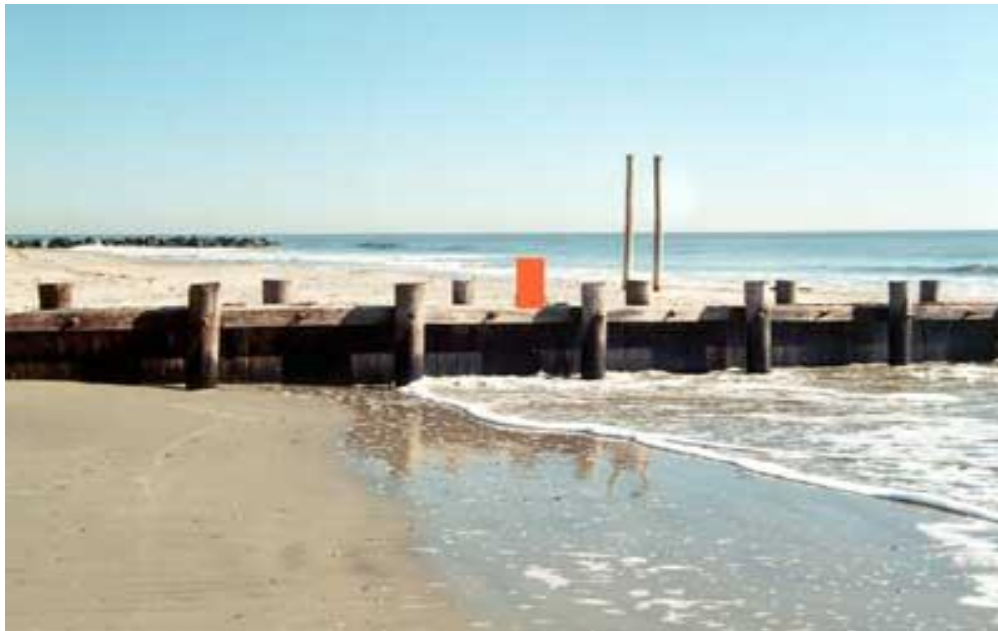
Fig.9.4: Photograph showing down drift of wood groin in the coast of Bluewater beach.
