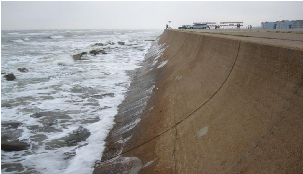
Fig. 9.7: Photograph showing vertical wall for protection of wave erosion in the coast.
