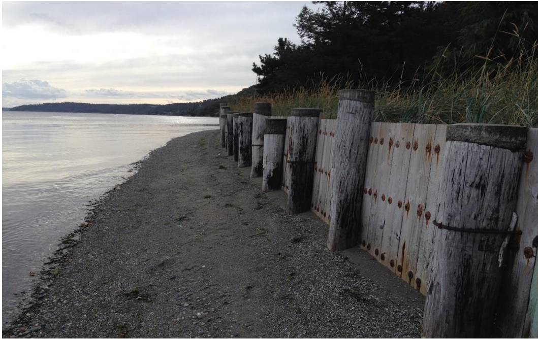
Fig. 9.8: Photograph showing bulkhead to protect bank erosion and slope failure.
