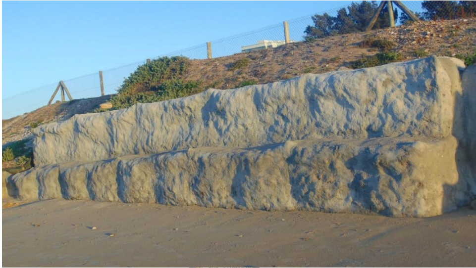
Fig. 9.3: Photograph showing cement hardening for protection of the bank in the Swartkops estuary.
