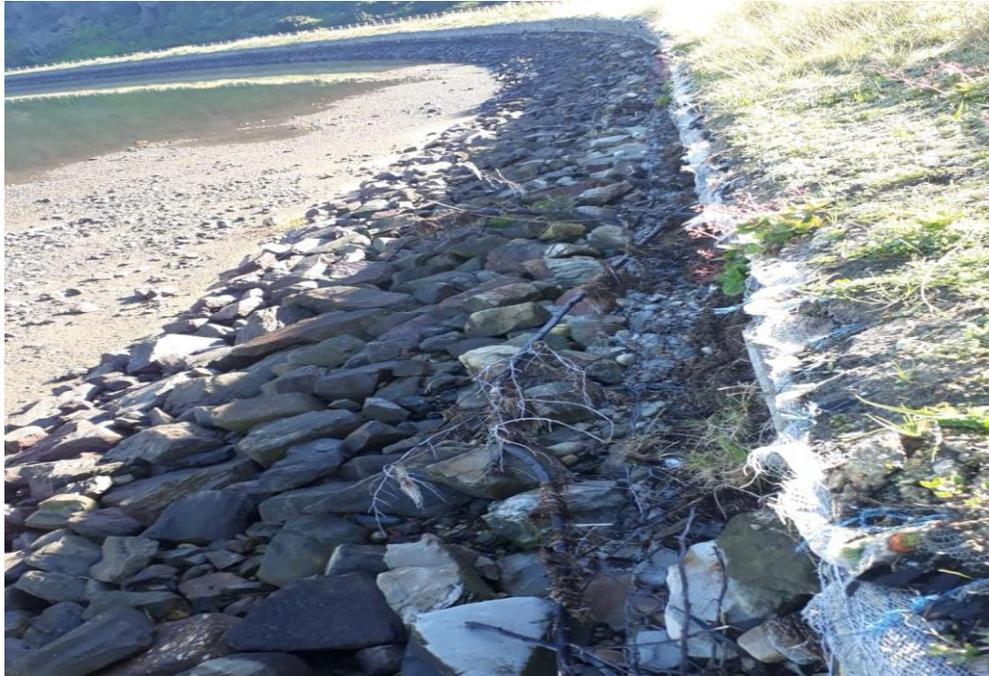
Figure 10.4: Photograph demonstrating riprap structures with pebble-and-boulder quartzite along the riverbank at Knysna.
