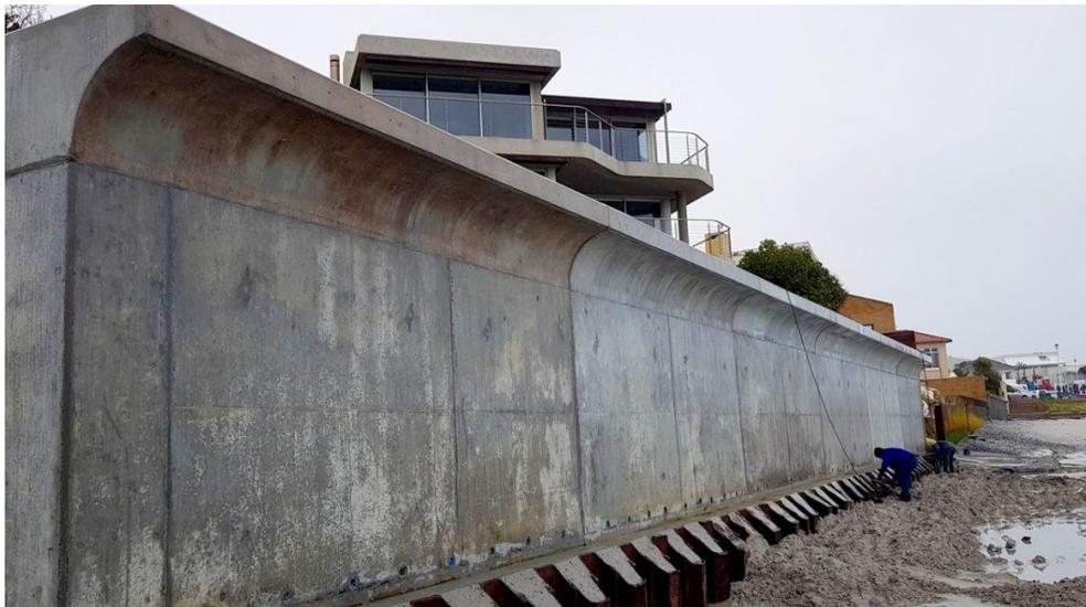
Figure 10.2: Photograph displaying a coastal seawall to protect infrastructures along Knysna Coast.
