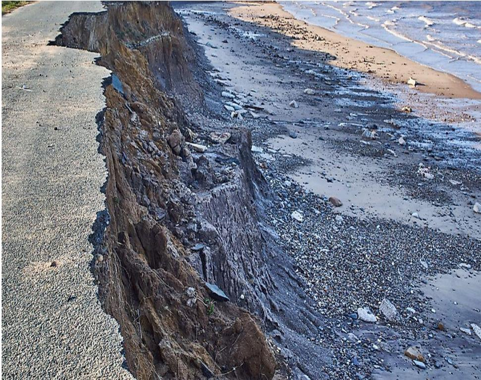
Figure 9.1: The photograph shows a tarred road washed away by water erosion in Durban.
