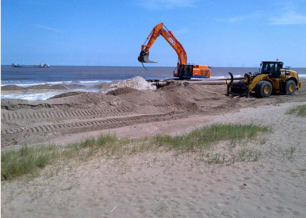
Figure 10.7: Photograph showing soft engineering solution (beach nourishment) to prevent flooding, Knysna in South Africa.
